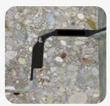
Centre the joint and assemble. The final position of the seal in the manhole joint is shown. If re-joinir is required, ensure the sliding skin is drawn bac to the position as shown the first picture.
