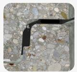
Centre the joint and assemble. The final position of the seal in the manhole joint is shown. If re-joining is required, ensure the sliding skin is drawn back to the position as shown in the first picture.
