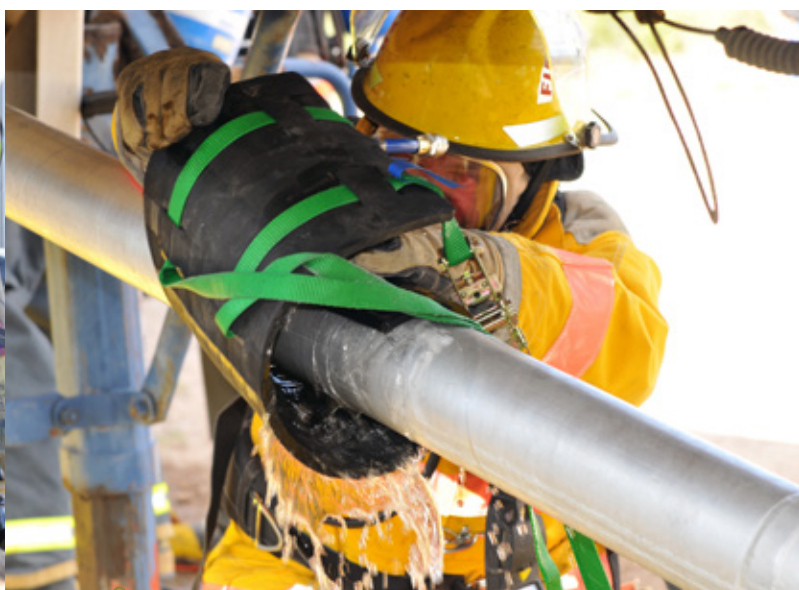
Pipe sealing
