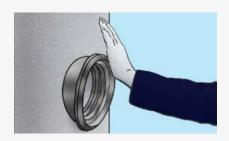
Press the seal into the hole. Do not use lubricant.
