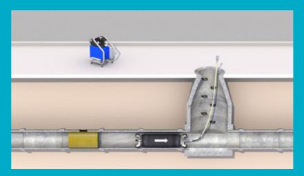
The resin-impregnated fiberglass mat can then be cured at ambient temperatures according to the information provided in the method statement or technical data sheets. The required cure times depend on the climatic conditions within the sewer. After the resin is completely cured, the packer is deflated and removed from the pipe.
