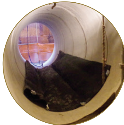
Placing – pillow plug should be positioned horizontally
