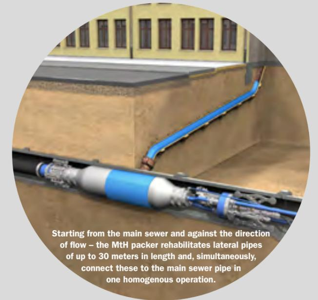
Starting from the main sewer and against the direction of flow – the Mth packer rehabilitates lateral pipes of up to 30 meters in length and, simultaneously, connect these to the main sewer pipe in one homogenous operation.
