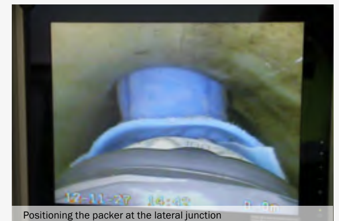
Positioning the packer at the lateral junction
