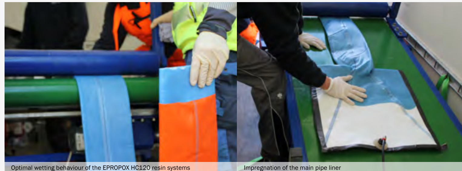
Optimal wetting behaviour of the EPROPOX HC120 resin systems
