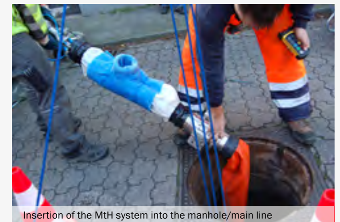
Insertion of the MtH system into the manhole/main line
