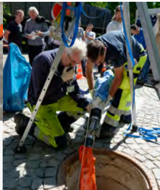
All system components of the Mth system are designed to pass through a standard manhole cover of 600 mm [approx. 23.6"] in diameter. The packer, for example, features an articulated joint which can be locked/unlocked at the press of a button. This ensures the smooth introduction of the packer into the main pipe even under confined conditions.
