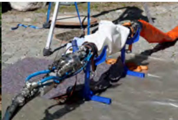
All system components of the Mth system are designed to pass through a standard manhole cover of 600 mm [approx. 23.6"] in diameter. The packer, for example, features an articulated joint which can be locked/unlocked at the press of a button. This ensures the smooth introduction of the packer into the main pipe even under confined conditions.
