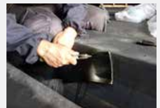
Apply compound layer
