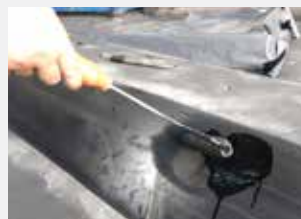
Apply bonding cement
