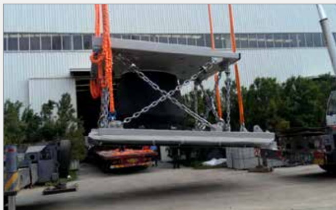
Handling of fender system using rigging equipment with spreader beam
