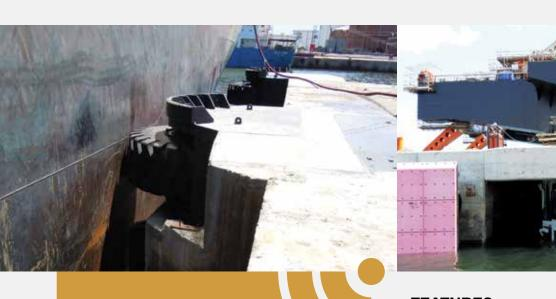
Wheel fenders are widely used on exposed corners to help ships maneuver into berths and narrow channels such as locks and dry-dock entrances.
