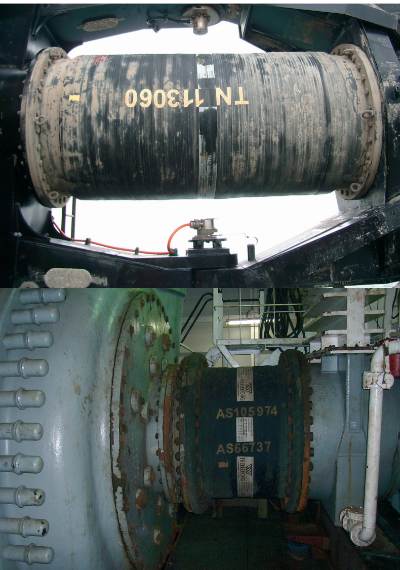
▲ Expansion joint in pumphouse
