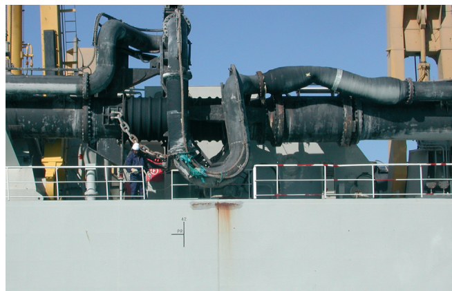
Suction and jetwater hose in trunnion joint suction pipe ▶
