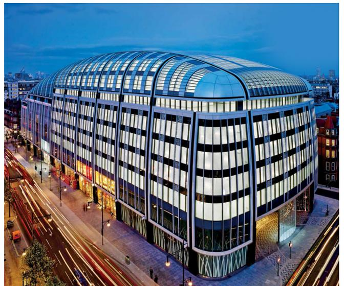
There are several hundred smaller bearings, 110 mm diameter, installed at the first floor level to isolate the exterior triple glazed cladding panels, which are suspended from a steel ring-beam at the level above.
