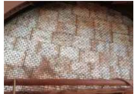
Spill face sloping walls and loading chutes
