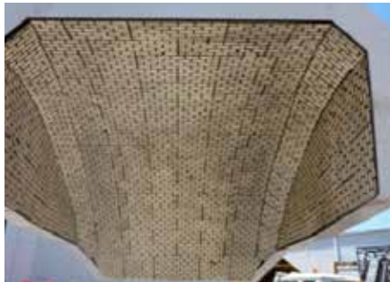
Completed re-designed deflector ready for service
