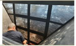
Depending on the application requirement, Hookgrip needs to cover between 20-40% of the total surface.
