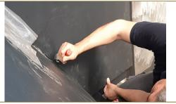
Once the rubber plate is placed in the correct place, press on the whole surface. You can use a roller for this purpose.
