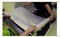
Put a plastic layer on top of the Hookgrip surface as in the picture to avoid direct contact between the hooks and the velour before the final installation.
