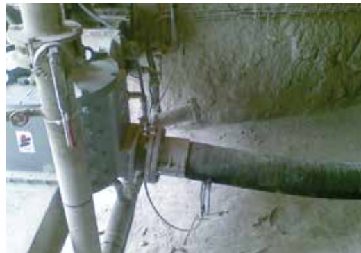
Micro-silica conveying 1 silo feeds 5 separate lines.
