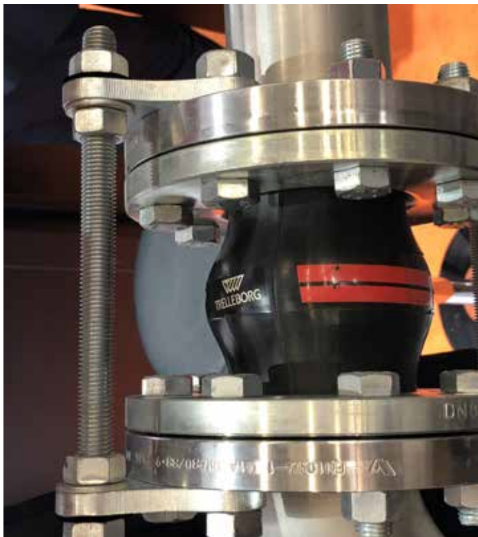
Expansion joint with tie rods blocking axial extension
