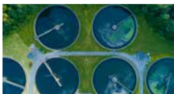
WATER & WASTE WATER MANAGEMENT
