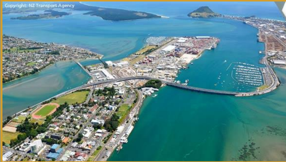
Chapel Street Viaduct, Tauranga Harbour Link, New Zealand
