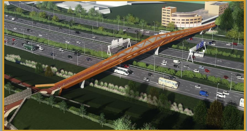
Trekietsviaduct (The Netherlands)
