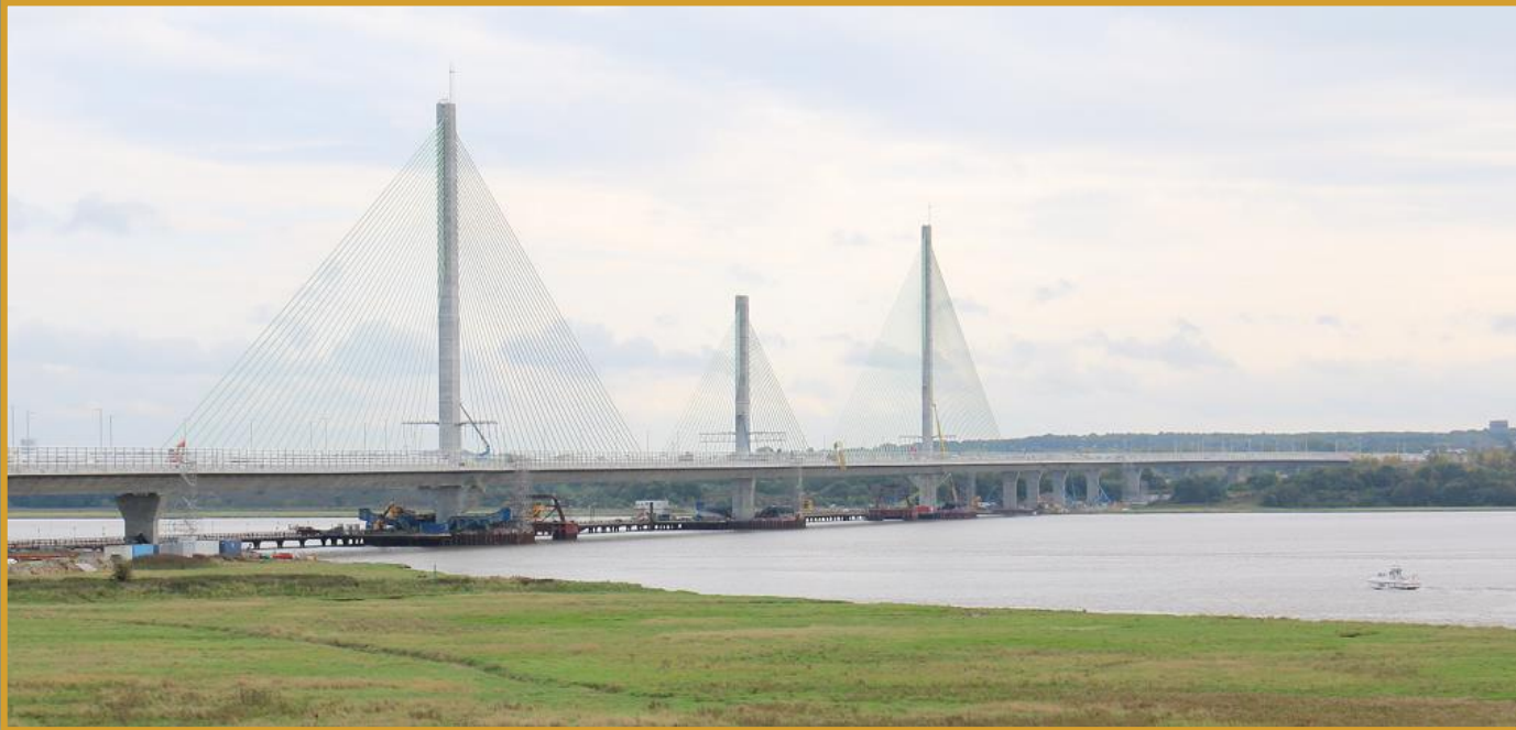
Mersey Link Bridge Liverpool (UK) 2,5 Km
