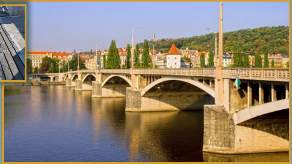
Jirasek Bridge Prague (Czech Republic)
