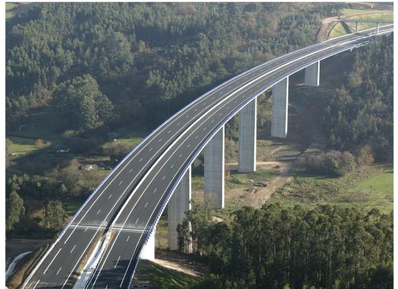
*The merge point between deck and road is one of the weakest points of modern steel and concrete bridge structure. A proper bond is key to bridge life. The system selected must provide a solid bond, enable transit of persons and vehicles; but at the same time allow for certain movements for the structure to adapt to the environment and thus endure with time.*
