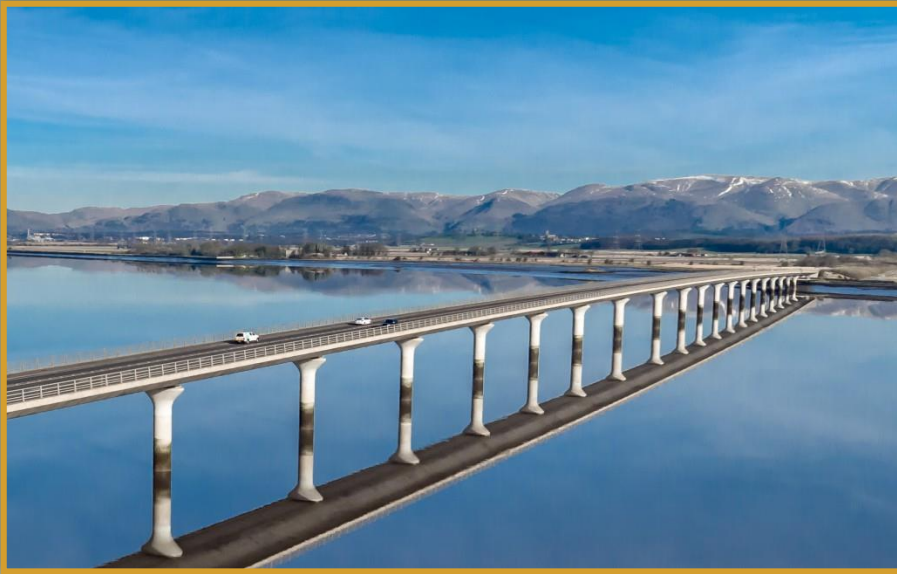
Clackmannanshire Bridge (UK)
