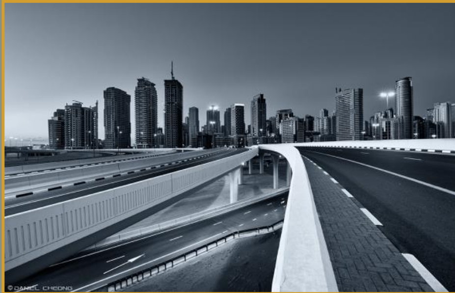
5.5 Interchange Dubai (UAE)
