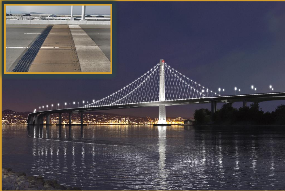
San Francisco Bay Bridge (US)
