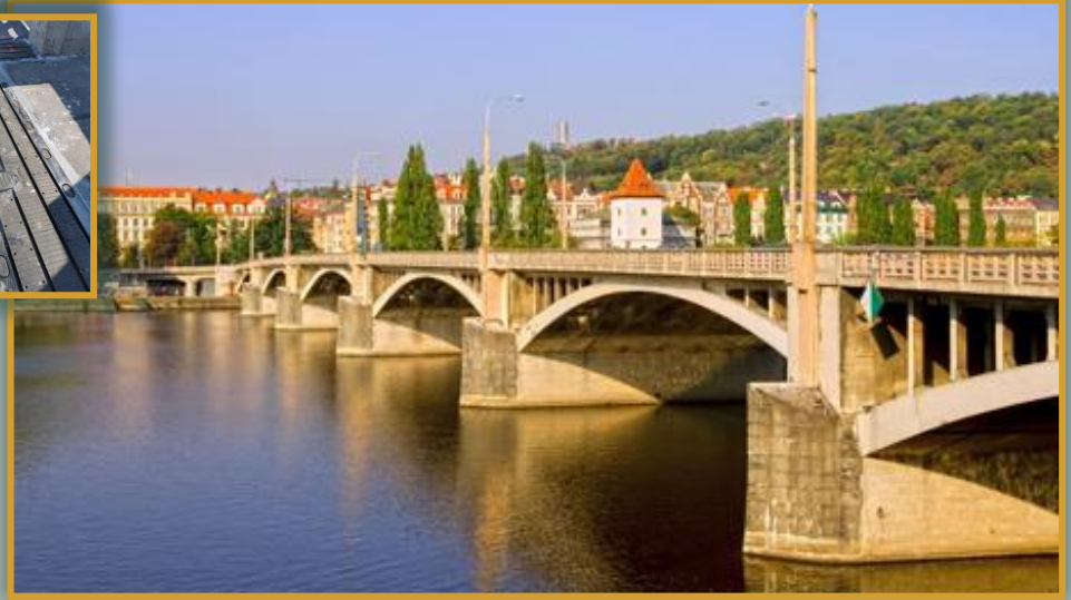
Jirasek Bridge Prague (Czech Republic)
