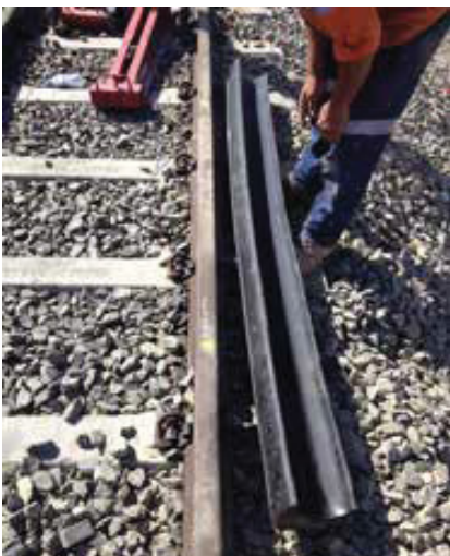
.....➤ Step 1 Position RX section in installation location
