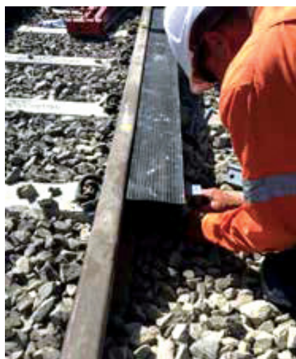
.....➤ Step 2 Position and loosely tighten retention brackets
