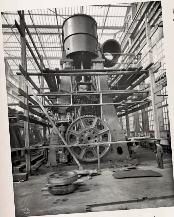
The port side engine of the Titanic under construction in Belfast, Northern Ireland. Source: Trustees of National Museums Northern Ireland
