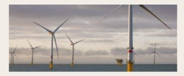
working on involves 62 by 15 MWh turbines, in total 930 MWh. This equals the annual use of electricity for 150,000 households.
