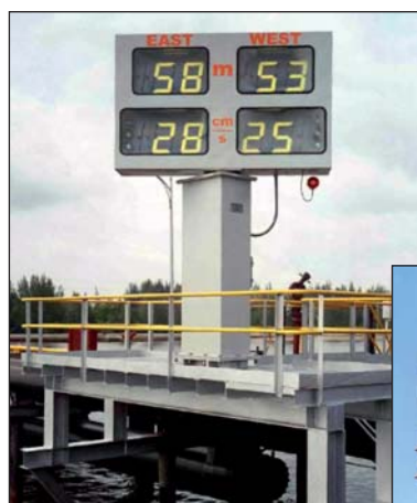
Display board on remote operation rotating pedestal
