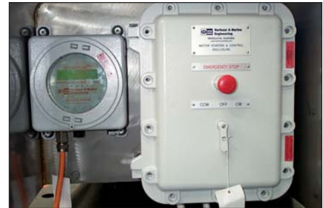
SmartHook® Local Display and Capstan Control Enclosure
