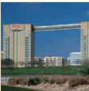
Skywalk bridge - Dubai EAU 2003
