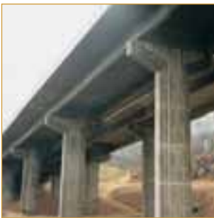
Gabalwia & Khiniza bridge EGYPT 2002
