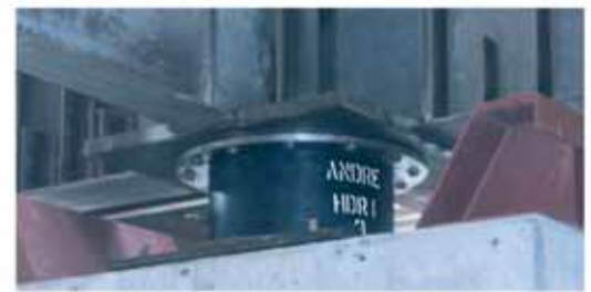
Andre High Damping Rubber Base Isolation Bearing installed under a ground floor beam of a 911 Emergency Operations Centre.
