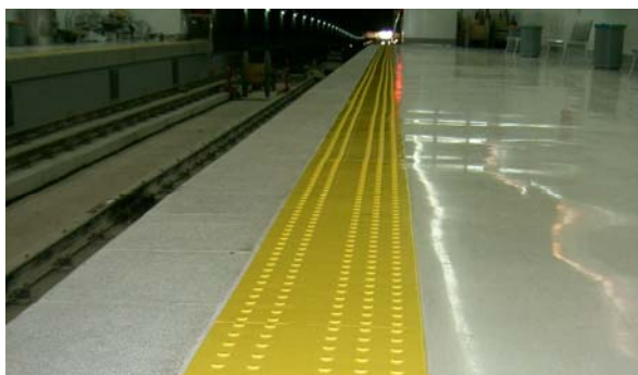
P. de Mallorca underground, platform edge
