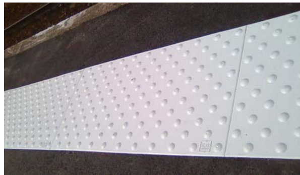
Platform edge SNCF, France
