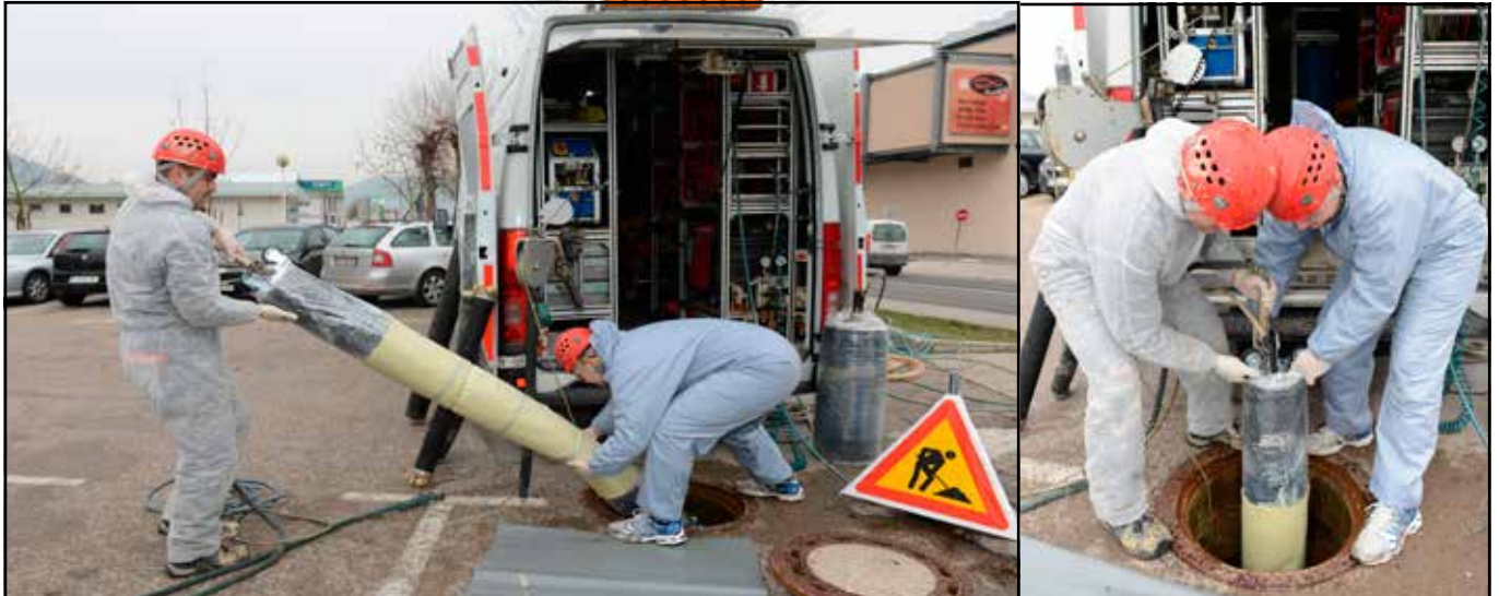
Figure 10: Insertion of SAVA packer into the pipe
