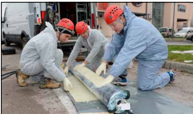
Figure 9: Application of resin-soaked fibres on the protected SAVA packer
