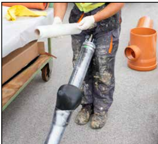
Figure 14: Fix the hat on the SAVA packer with foil
