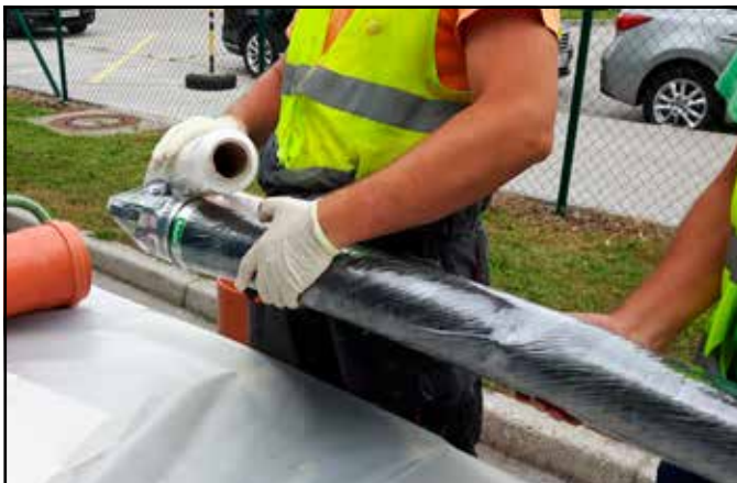
Figure 11: Application of protective foil on SAVA packer
