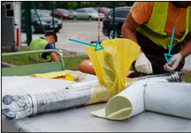
Figure 16: Apply PVC protection on the hat
