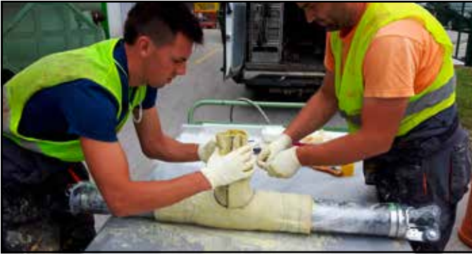
Figure 18: Apply resin-soaked fibres onto the protected SAVA T packer and fix them with rubber bands
