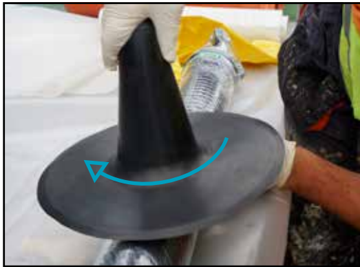
Figure 13: Screw the hat on the SAVA packer Figure 13: Threaded insert M6
