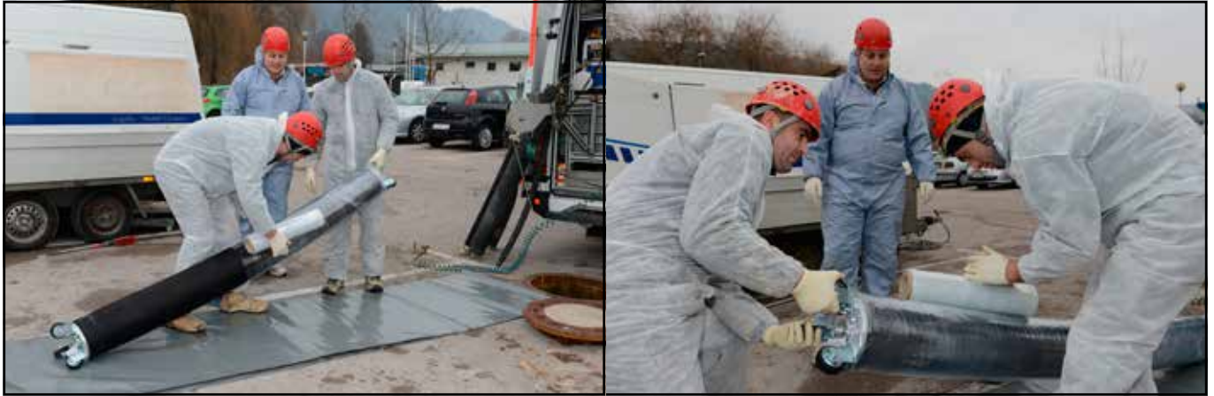
Figure 8: Application of protective foil on SAVA packer
