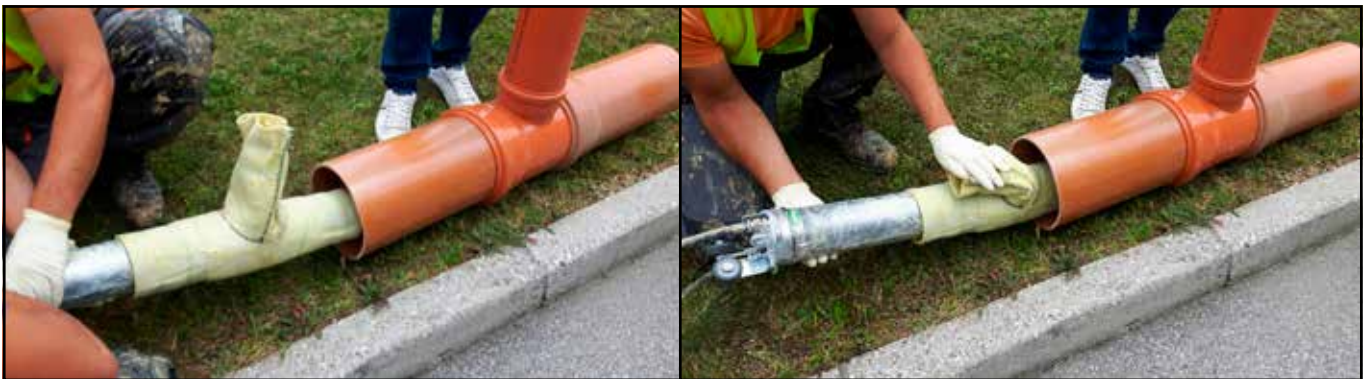
Figure 19: Insert the SAVA T packer into the pipe
