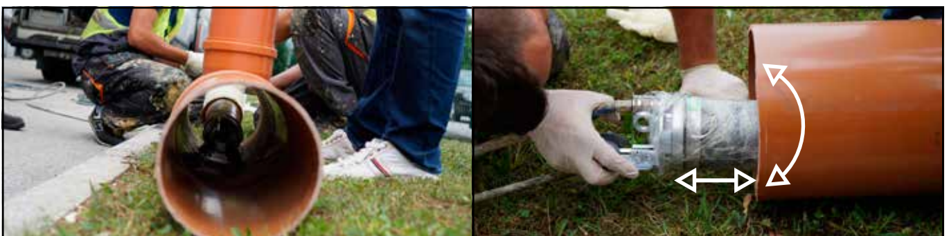
Figure 20: Insert the SAVA T packer into the pipe and position it
