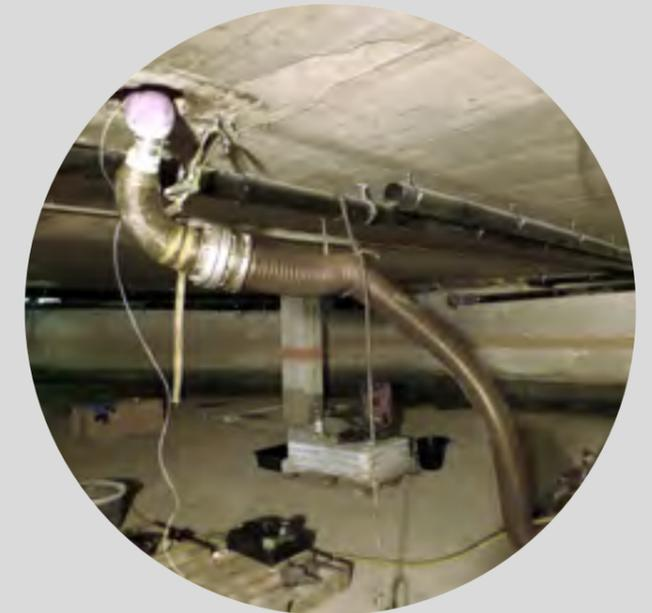
would pose challenge for the installers as it included two 45-degree bends and another two 90-degree bends over a distance of 13 metres, 7.5 metres of which were vertical. The team also performed a pressure test.
