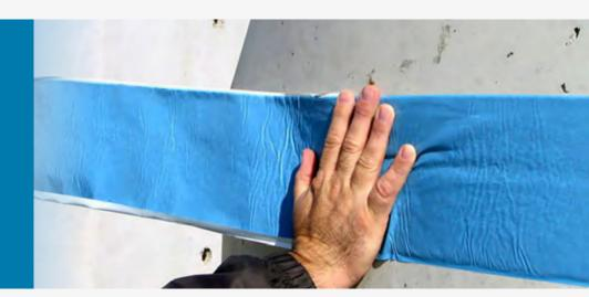
External Joint Wrap is a custom compounded butylbased sealant specifically designed to create a high performance seal in precast structures and pipe joints.
