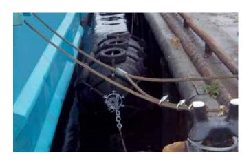
"The docking of the accommodation vessel demanded a high quality fendering system capable of providing a safe and reliable cushion between the vessel and quay for the duration of both industrial projects."
