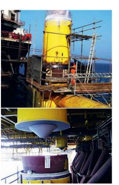
Using LMUs during a float-over process, the loads can be transferred from the barge to the base structure in a controlled manner. LMUs consist of a steel structure incorporating rubber elements to achieve a specified spring rate, depending on the expected loads and movements.
